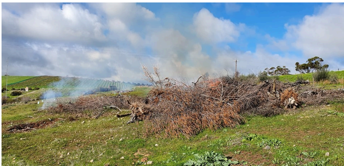
Image: Olive trees being burnt at the Quarry Road Dam site, McLaren Vale SA
